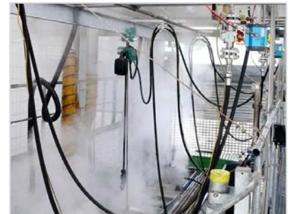
Operational area tank cleaning: JDN Air Hoist PROFI 05 TI in manual trolley.
